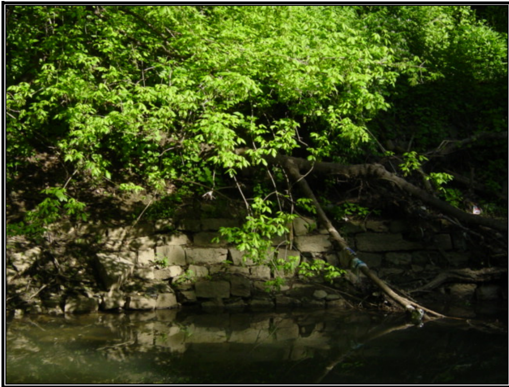
Figure 6.16. Stone wall along west bank of Beargrass Creek, looking northwest.
