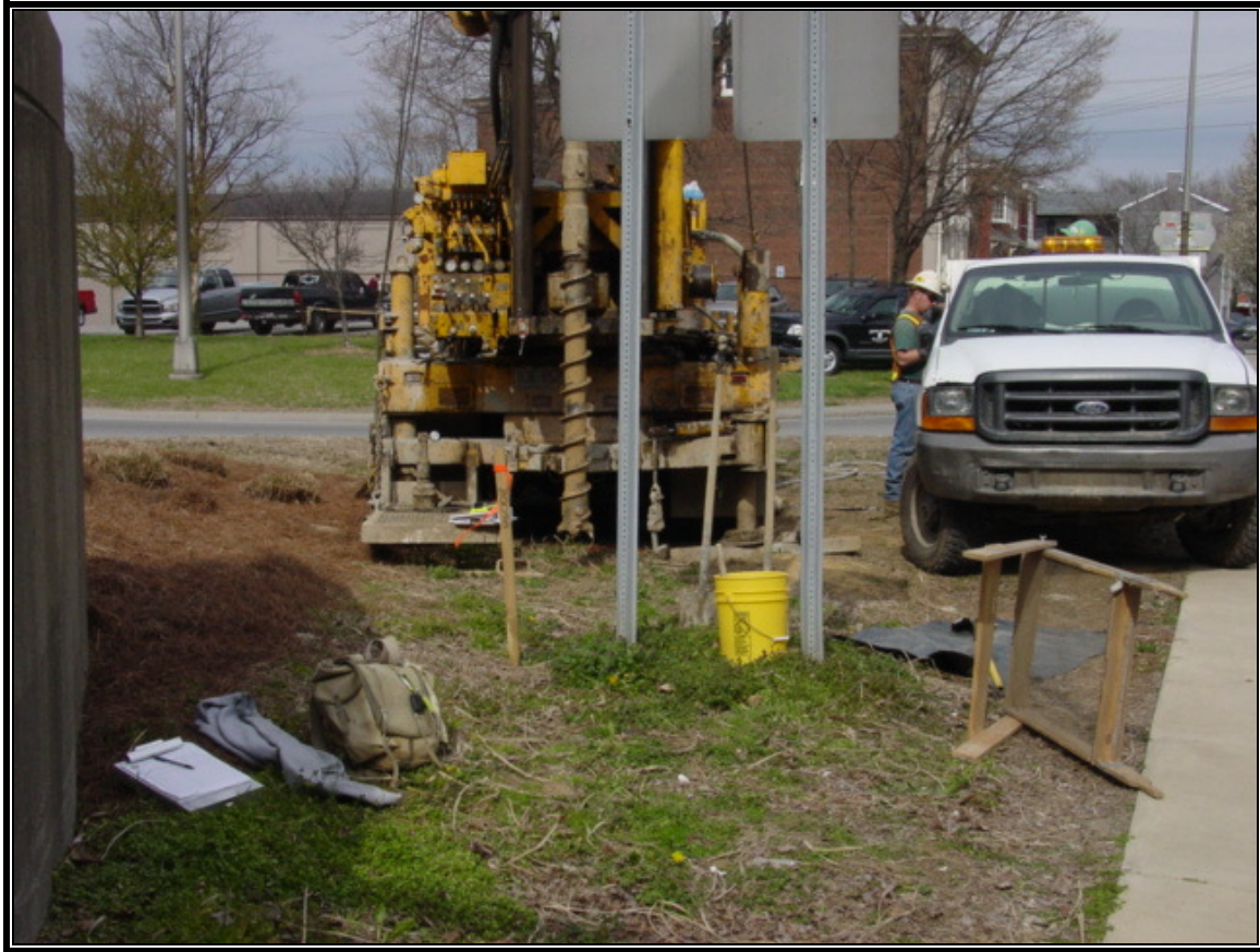
Figure 4.1. Drill crew augering a bore hole.
